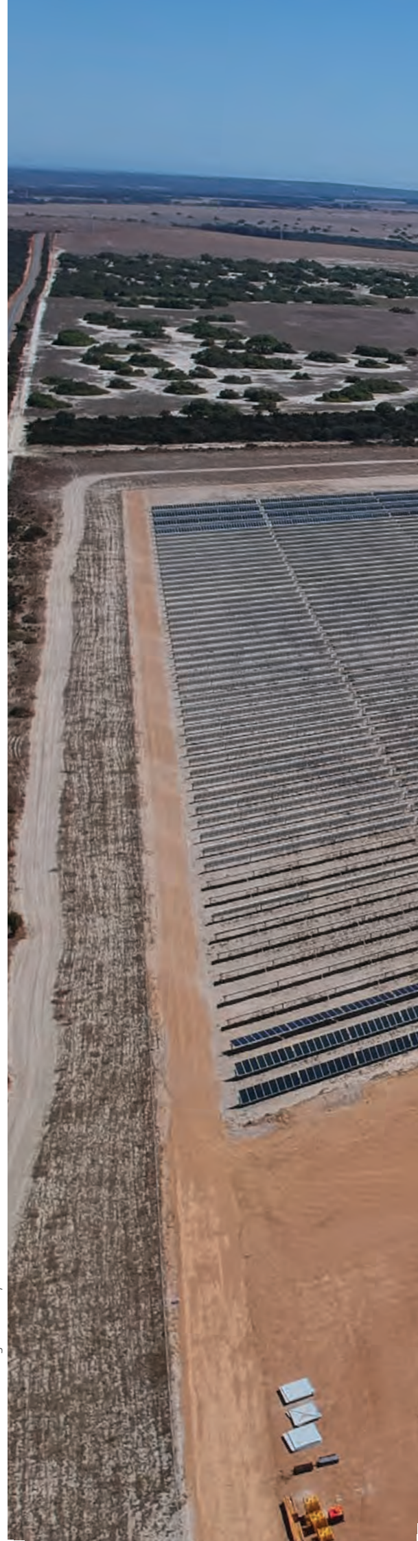
Emu Downs Wind Farm. Image courtesy of APA
