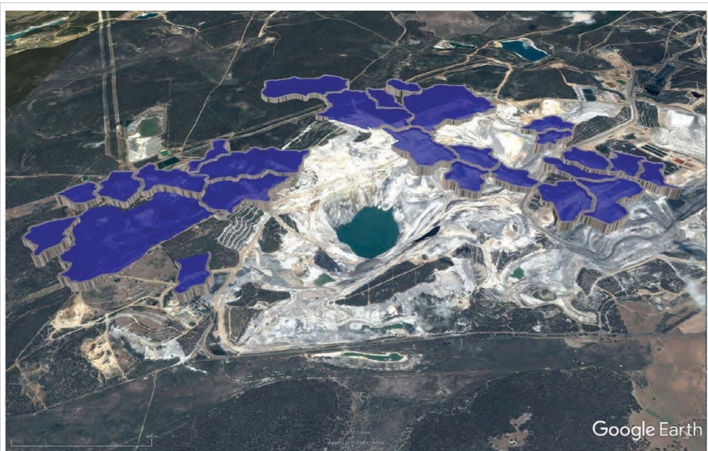
Figure E.1 Conceptual Pumped Hydro installations in repurposed Collie coal mines. Image sourced from A. Blakers et al. (2018).
